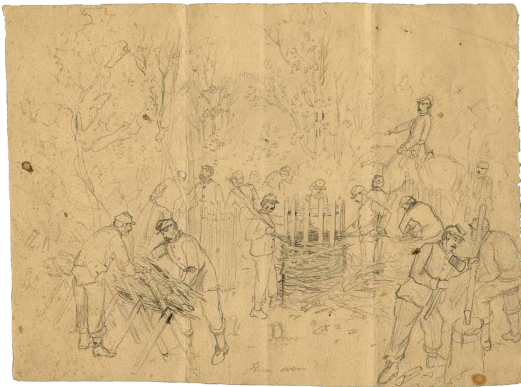
101. Francis H. Schell, Making Fascines and Gabions in Kentucky , 1863. Graphite on cream heavy gauge wove paper, 7.3 x 9.8 in. (18.5 x 24.9 cm). CW-FHS-KY-NDc
