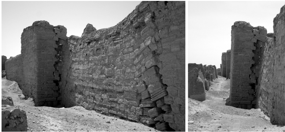
Figure 18.3: Damage to the city wall and Tower 19, as seen in 2008. The undermined stretch of wall came “unzipped” at each end and sank into the ground, as did two walls of Tower 19. These were kept upright by the earth rampart that then enshrouded them, which was removed by Du Mesnil during the excavations (photograph by the author)
