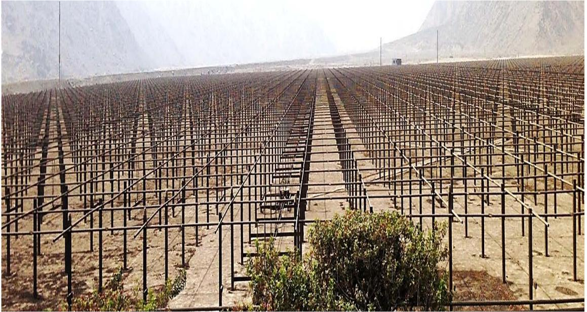
Figure 3.1: The main radar antenna in Jicamarca Radio Observatory (JRO), Peru, one of the largest of all the incoherent scatter radars (ISRs) in the world where the magnetic dip angle is about  $1^\circ$ . The main antenna consists of a 300m x 300m square array composed of 18,432 cross-polarized dipoles.
