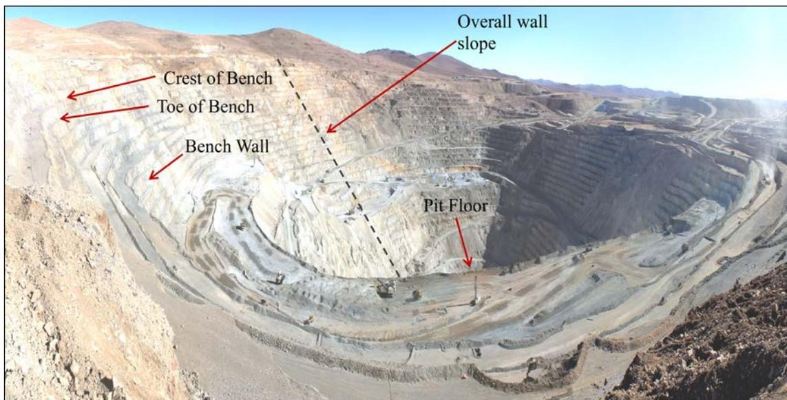
**Figure 1.1:** An image of a typical open-pit mine with main parts labeled. (Urzua, 2012).
